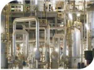
Water Piping System
